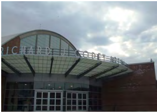
New development in the Saint Cloud commercial area should leverage Codey Arena and other Essex County facilities.
