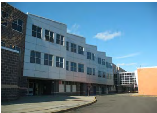
West Orange High School was recently upgraded and expanded.
